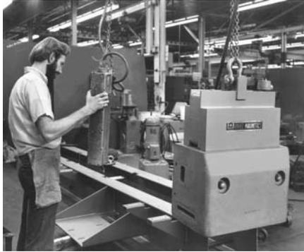
Specifically designed to provide greater contact and holding strength on castings, forgings, plates and structural shapes
